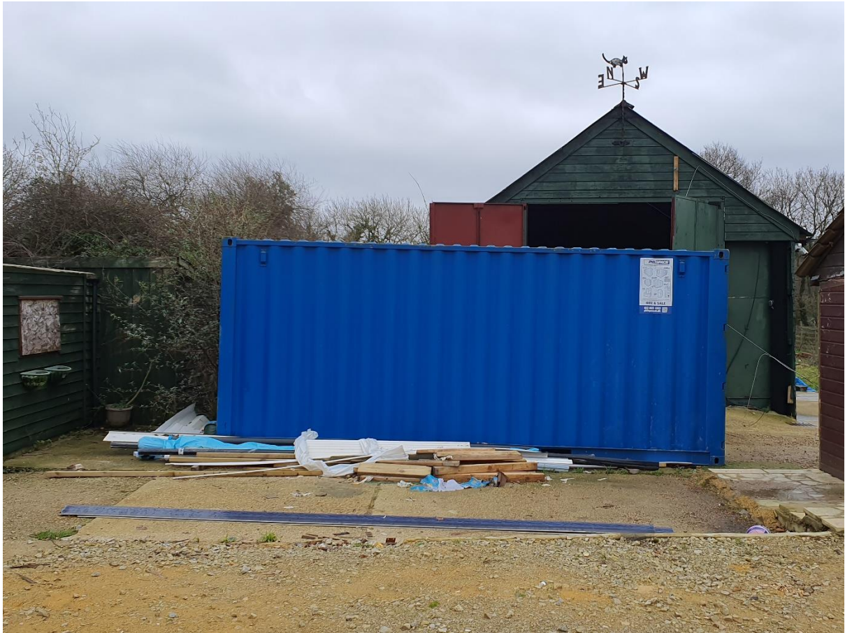
NW Gable of barn behind blue structure_20210119_145056.jpg
