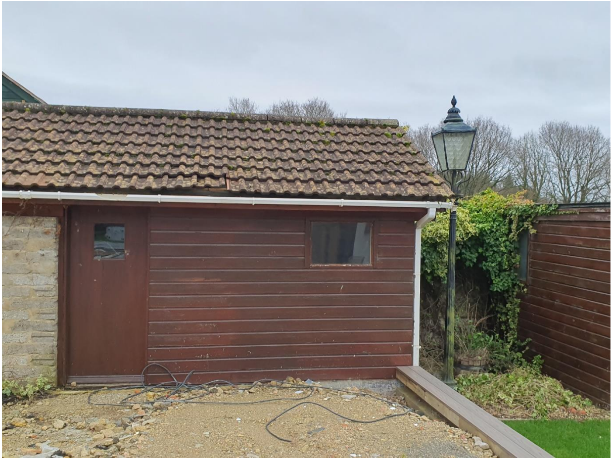
NW Gable of barn behind bldg_20210119_145106.jpg
