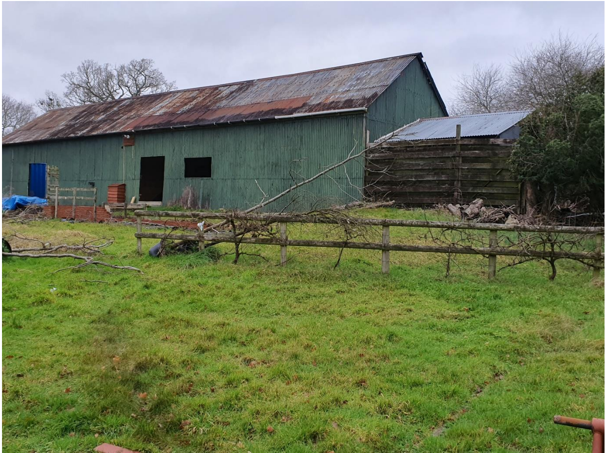
SW Elevation (end gable is SE elev) - 20210119_144830.jpg
